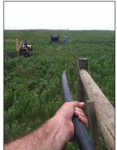
The first additional level of permanence is to use welded couplings with an above ground HDPE pipe system instead of removable compression couplers and fittings. Wayne Vincent with Common Sense Manufacturing of Faulkton utilizes welded couplers on many of their overland water systems.
